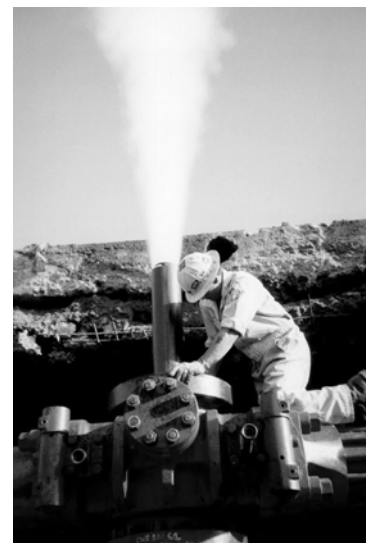
Figure 3-21: Well capping operations (on land, temperate)
