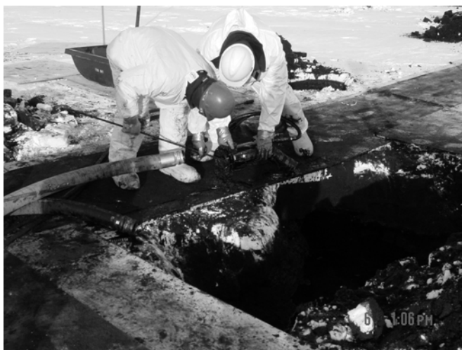
Figure 4-2: Cleanup operations for a pipeline spill to tundra on the Alaska North Slope (ADEC 2006)
