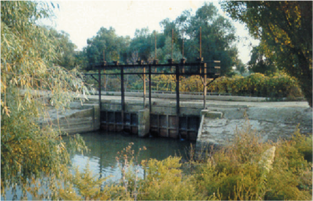
Figure E.6 A sluice on Skunda canal (view from lake Kugurly)
